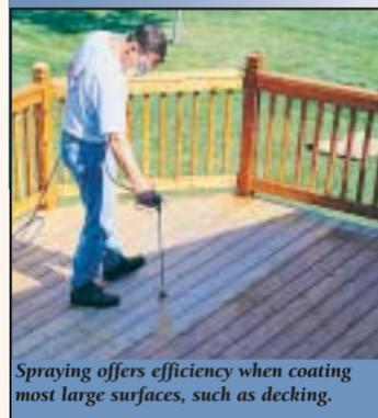
Spraying offers efficiency when coating most large surfaces, such as decking.
