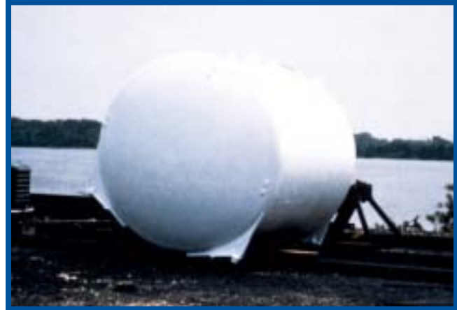
Tank after topcoat application.
