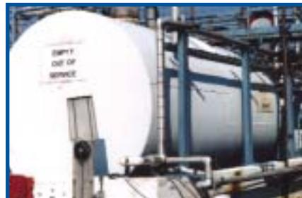
Typical tank painted with an all WB system after 12 years exposure.
